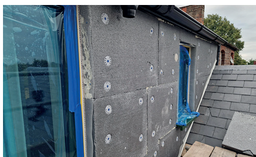
External view of our second floor bedroom after new windows and external wall insulation was installed over the solid brick wall, prior to rendering.
