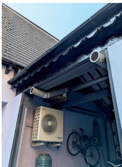
Grant (air source heat pump), and the vents to Paul (internal mechanical ventilation)
