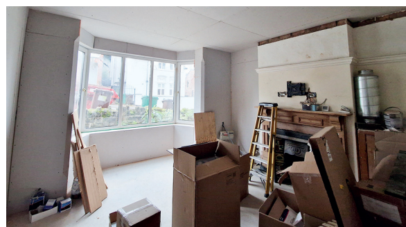
Our front room after internal insulation was added to two walls and the underside of the bay roof, followed by plasterboard, prior to plastering. Underfloor insulation and heating were also added to this room, and the whole ground floor, with a new concrete subfloor.
