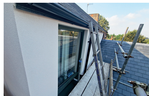
Our second floor bedroom exterior wall and windows after rendering over the external wall insulation.
