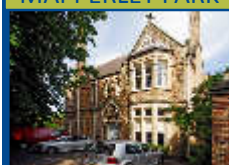
MAPPERLEY PARK Cyprus Road 2 bedroom ground floor apartment with garage and large garden £250,000
