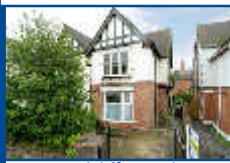
Redcliffe Road Potential 6 bedroom family home currently 2 apartments £195,000
